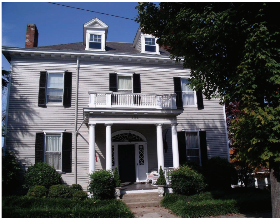
401 Washington Street-Long House (C. 1902)-Built for Armistead R Long as it appears in 2010.
